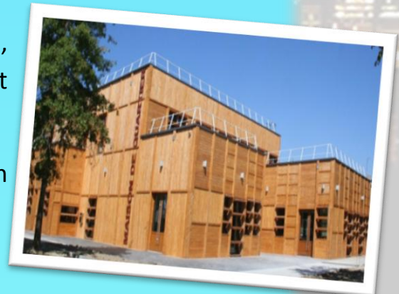
Neighborhood house Bottières in Nantes 19,4 % of electricity savings
