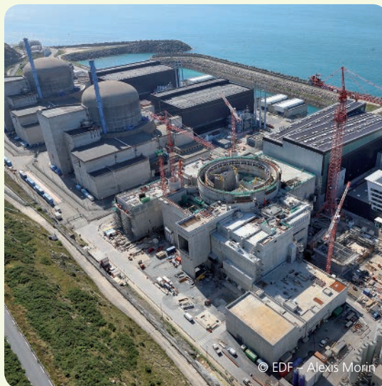
Flammanville 3 under construction
